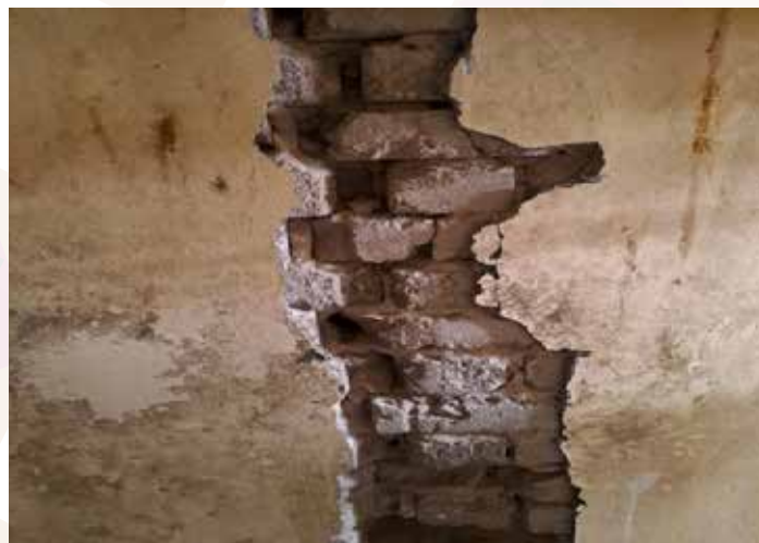
Cracked wall of the holding cell
